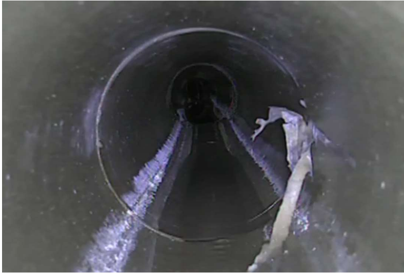
150 ft. Gasket Overpour at service line
