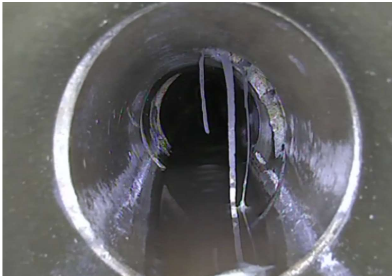
150 ft. Gasket Overpour at service line
