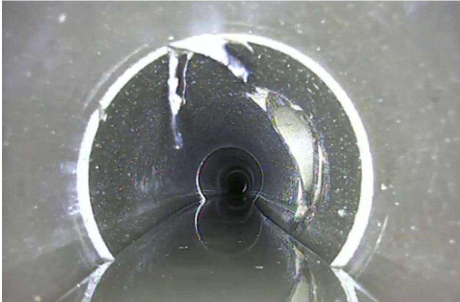
270 ft. High water line (Not a deficiency)
