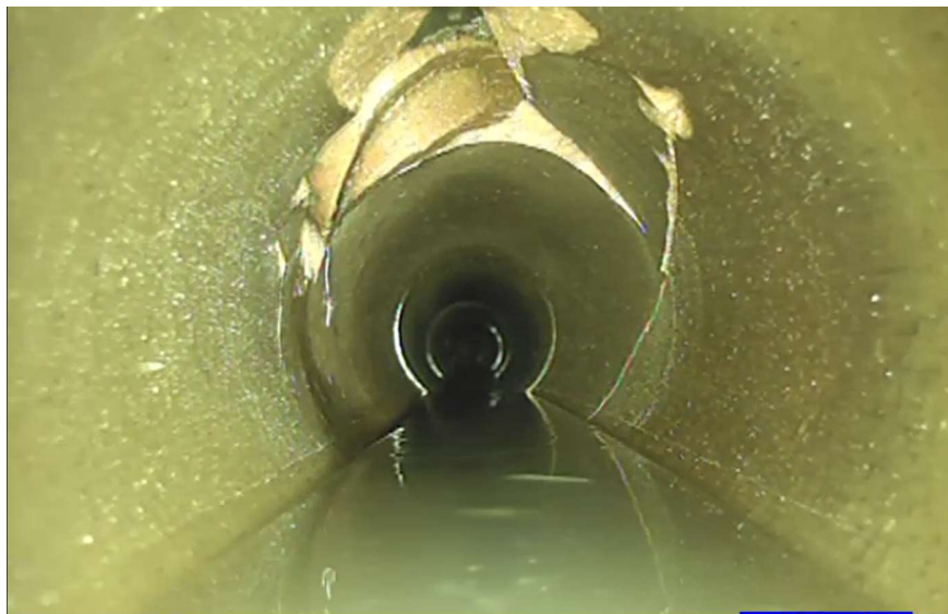
138 ft. Cracking/Broken
