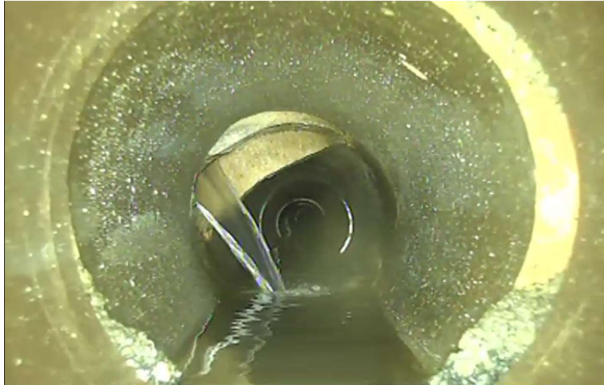
138 ft. Cracking/Broken
