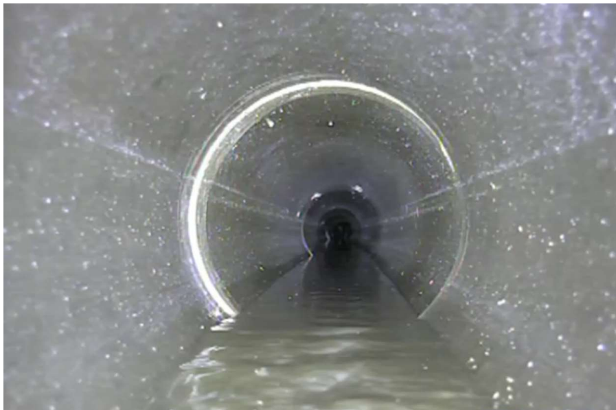
270 ft. High water line (Not a deficiency)
