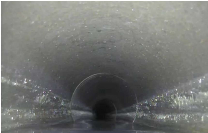
Video #7B 11 ft. Grease Build Up
