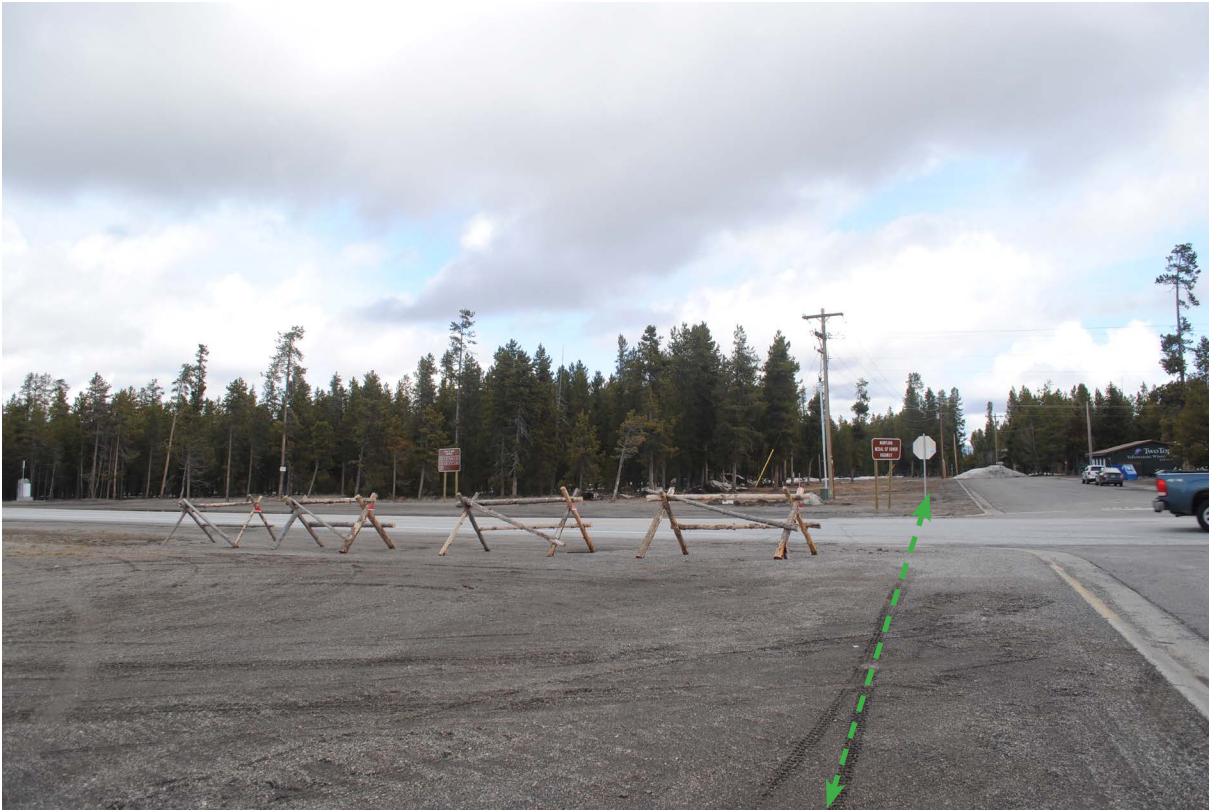
Figure 3.2. Intersection of Iris Street with US 20 (Targhee Pass Highway), looking north. The wood barricades on the center of the image were placed by the Town to deter drivers from cutting through the adjacent lot when highway is congested.
