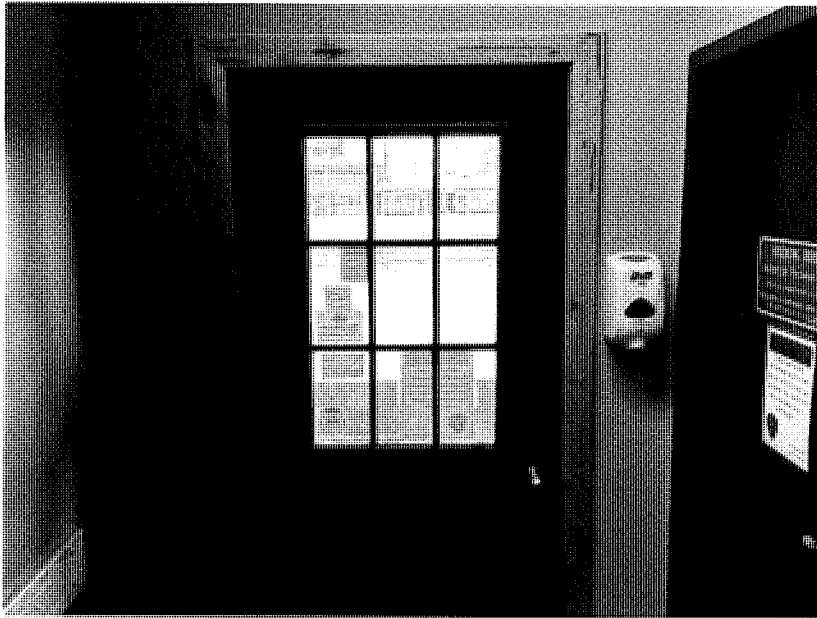
Current Interior of front door
