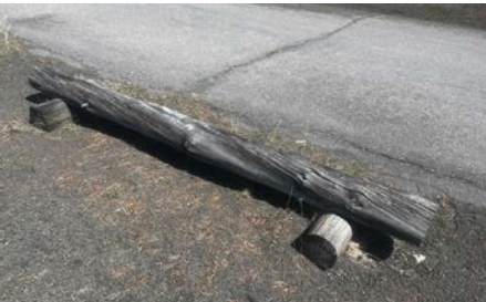
Log barrier to delineate shared path
