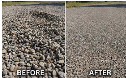
Compacted / infilled aggregate
